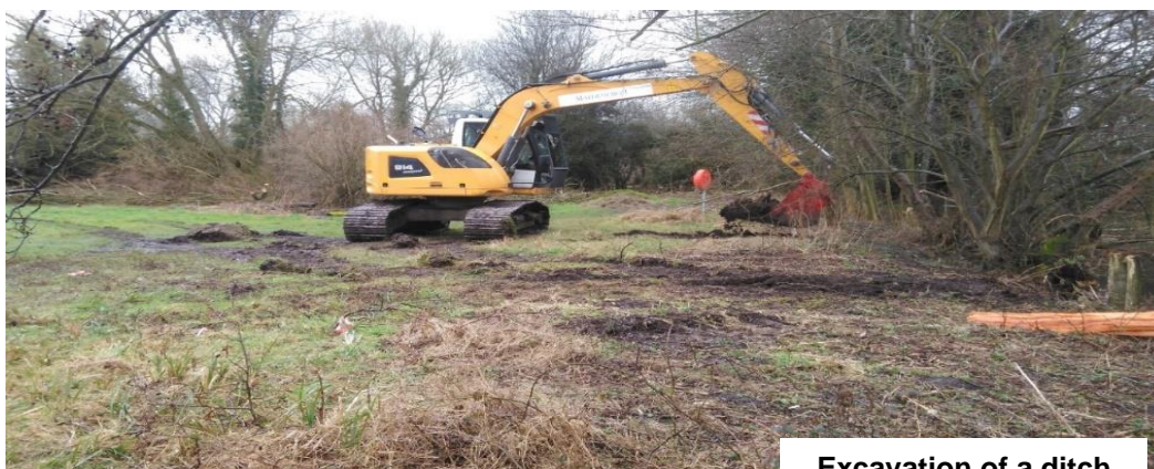
Excavation of a ditch
